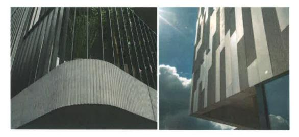
The POLYCON material is a composite material based on concrete, the basic recipe of which contains basic cement mass, fine aggregate, water, dispersed resistant glass fibers and other chemical additives. Thanks to this combination, the necessary technical properties are achieved, such as hardness strength, long life, fire resistance of class A1.
